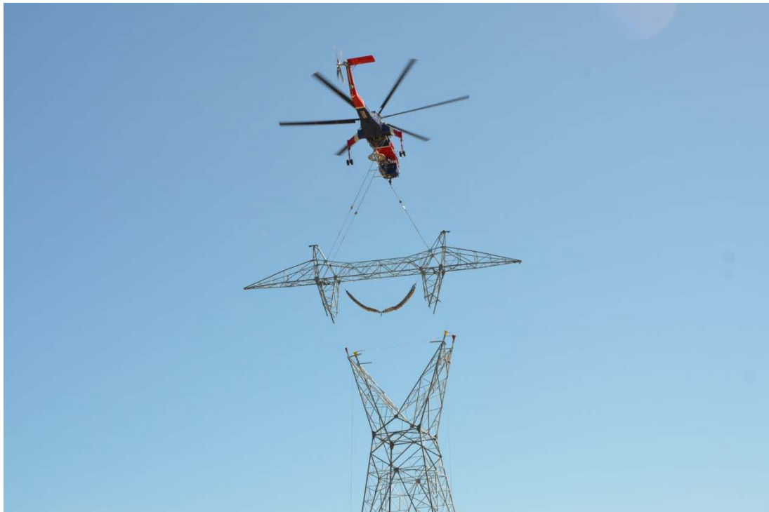
Air crane setting tower bridge on EP 218.
